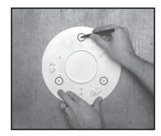
• Open the three mounting holes on the base and mark the holes to drill, pointing the arrow to the top.
